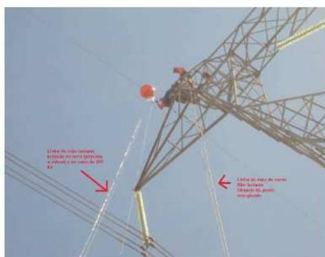
**Figure 6:** Placing signalization sphere.
