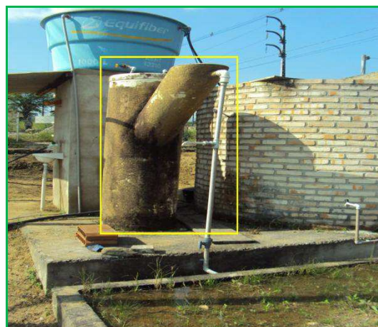
Figura 4. Reator UASB
