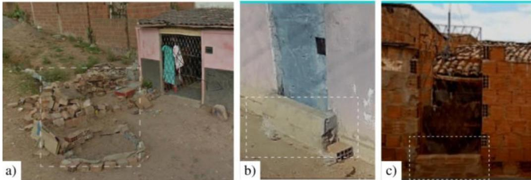
**Figure 3:** Improved barriers to protect households against the entrance of water during stormwater events. a) Rubble barriers, b) and c) Brick masonry barriers in the house's front door. Source: a) Google Earth [10], b) and c) Photos taken by the catchment's inhabitants in 2021
