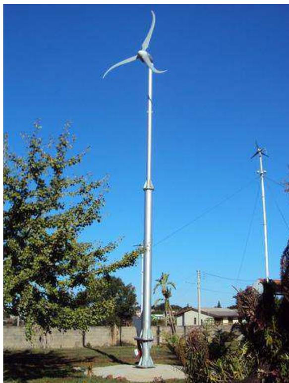
**Figura 14. Aerogerador *Skystream 3,7*.**
